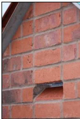
Figure 1: Habibat Bat Box faced with red brick, incorporated within wall at gable end.
